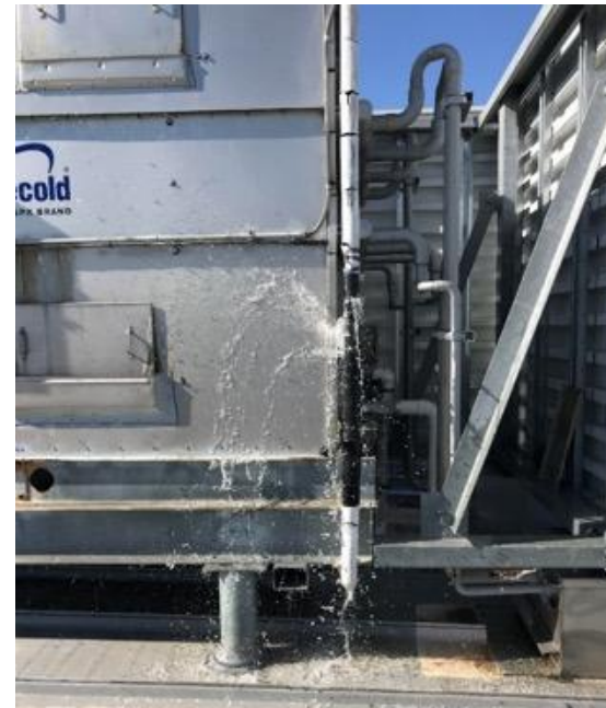
Example of a Water Leak and Overflow
