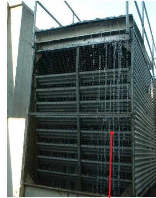
Example of a Water Leak and Overflow
