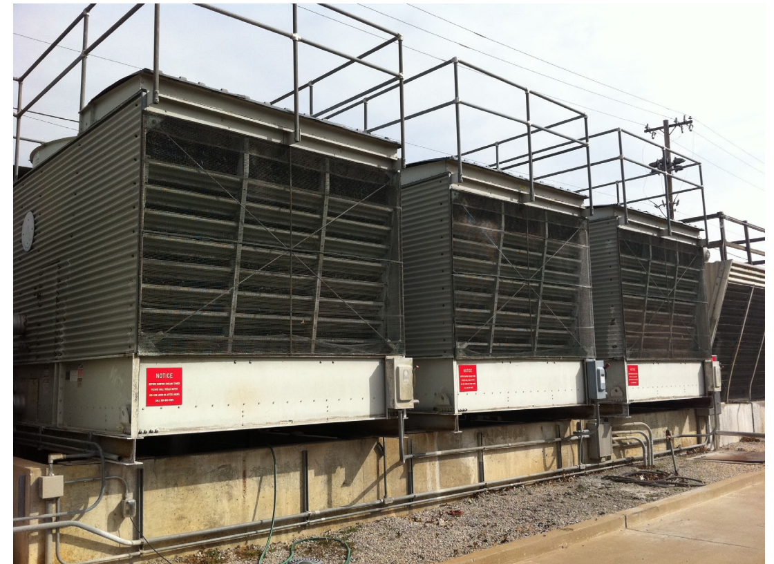
Water-Cooled Condenser Using Cooling Tower (Open Loop)
