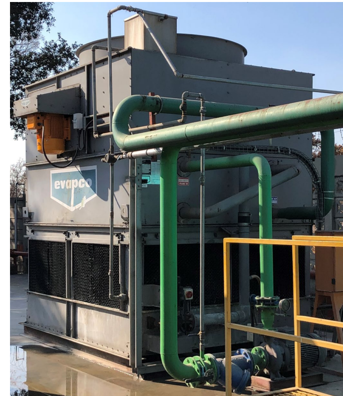
Water-Cooled Condenser Using Indirect Cooling (Closed Loop)
