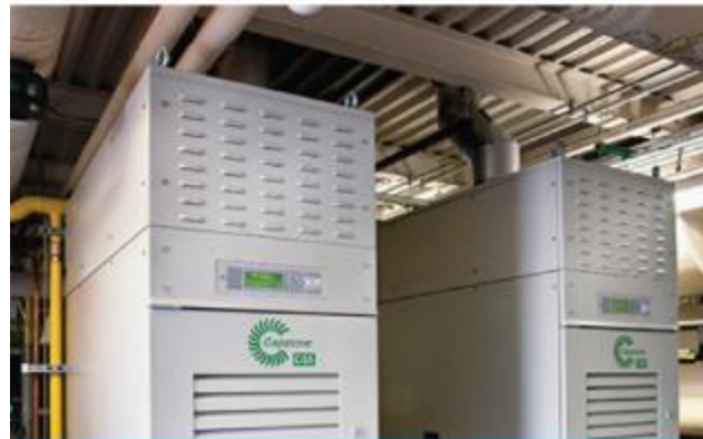
Microturbine CHP installation at a commercial facility. Photo courtesy of Capstone Turbine Corporation.
