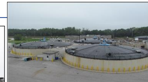
WPCP Anaerobic Digester Tanks (Photo Courtesy of WPCP)
