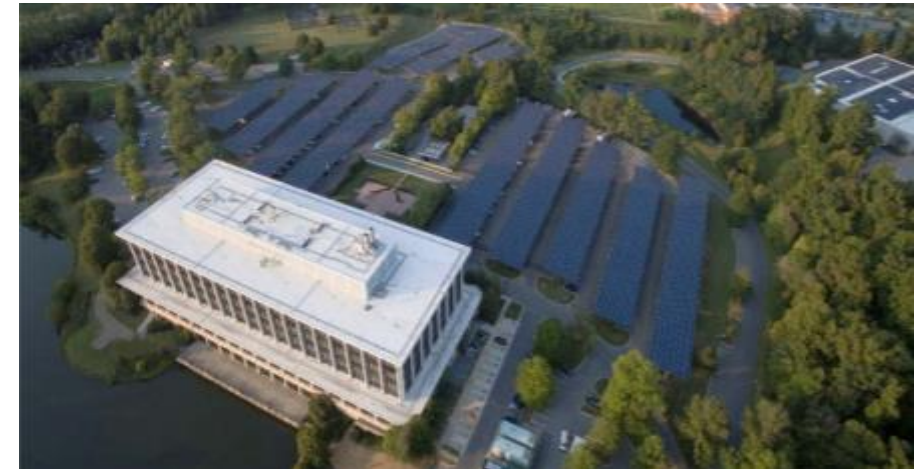
The CHP system is accompanied with 2 MW of solar capacity. Photo courtesy of Montgomery County.
