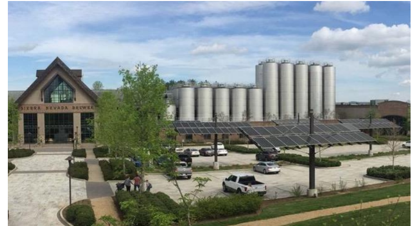
Sierra Nevada Brewing in Mills River, NC has 600 kW of solar PV and 400 kW of biogas microturbines (photo: DOE Onsite Energy TAP)
