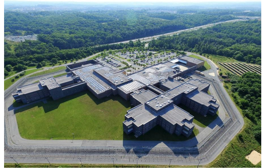
220 kW CHP system with 2.8 MW of solar PV capacity. Photo courtesy of Montgomery County.
