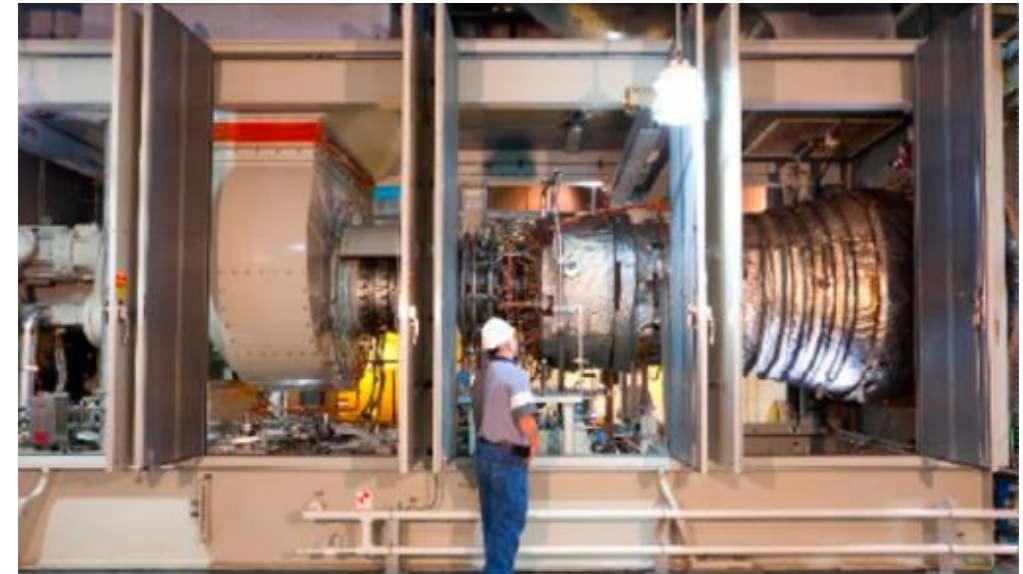
Gas turbine CHP installation at a university. Photo courtesy of Solar Turbines
