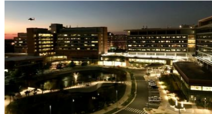
By using CHP, Shands hospital was able to achieve LEED Gold certification from the U.S. Green Building Council.
