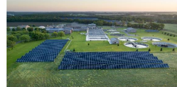
220 kW (left, installed 2017) and 240 kW (right, installed 2020) Solar Arrays Source: St. Cloud NEW Recovery Facility
