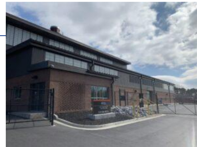
The Duke Energy owned and operated CHP system at Clemson reduces emissions by 49,000 MT CO 2 e annually.
