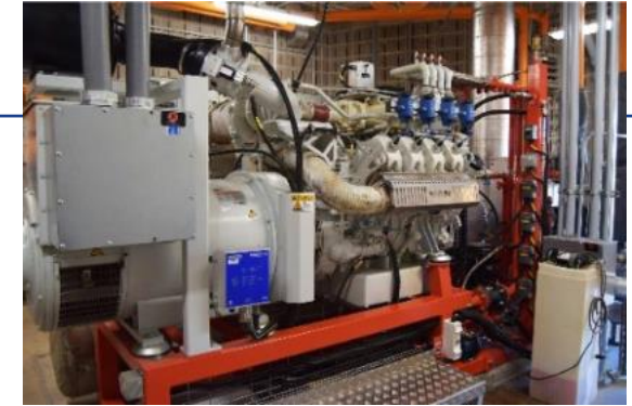
375kW CHP Engine/Generator Set Source: DGSD
