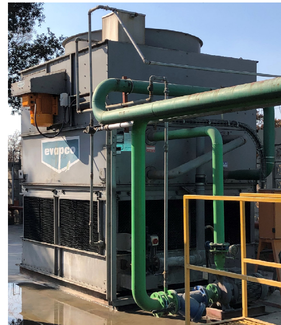
Water-Cooled Condenser Using Indirect Cooling (Closed Loop)
