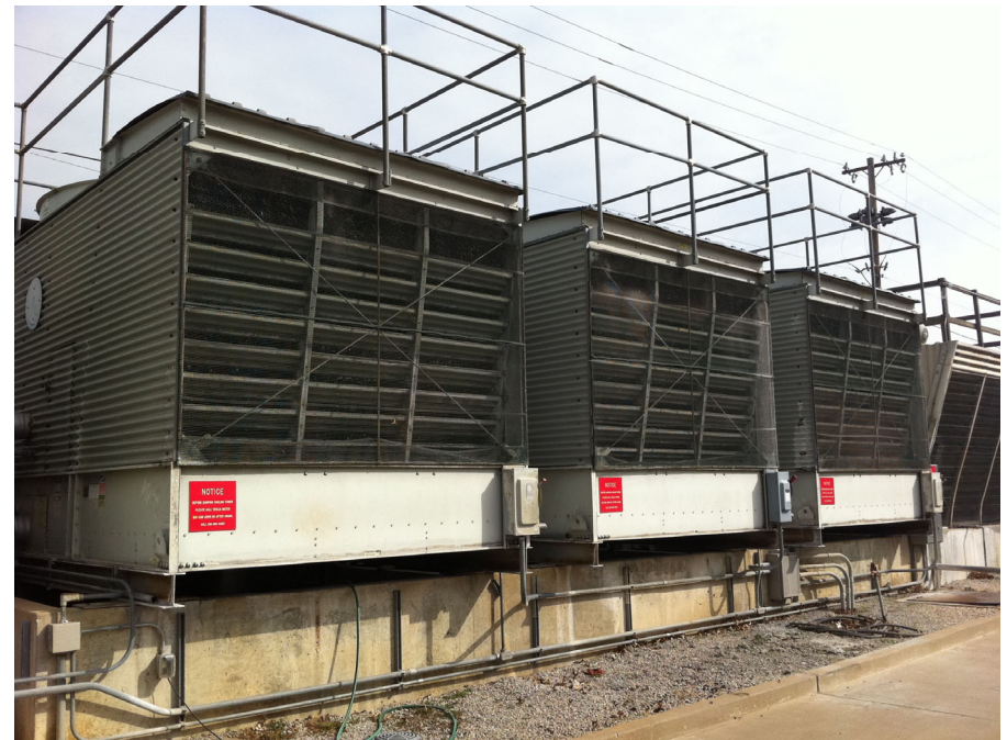
Water-Cooled Condenser Using Cooling Tower (Open Loop)
