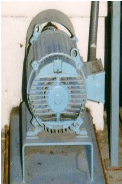
15 kW motor efficiency = 91%
