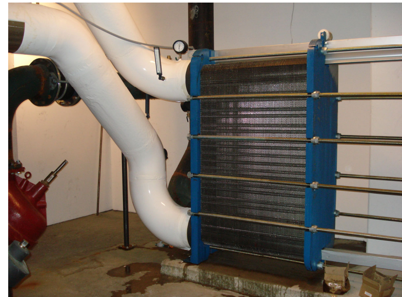
Plate and Frame Exchangers
