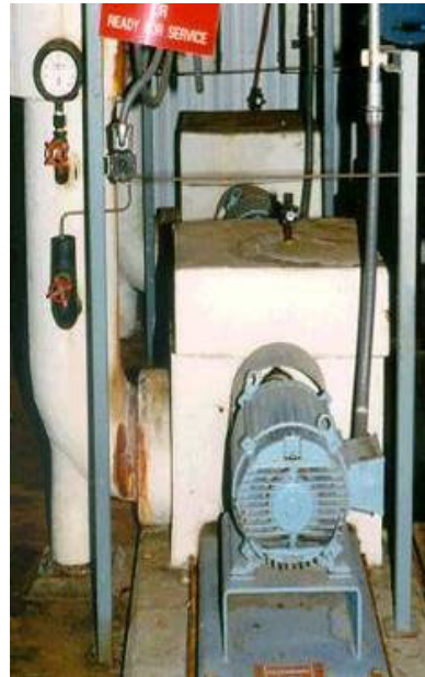
Combined motor & pump efficiency = 59%
