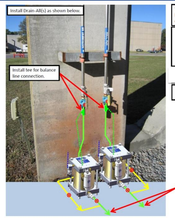
The orientation and location of the Drain-All trap should be adjusted to best accommodate piping and discharge direction to drain considering available space.
