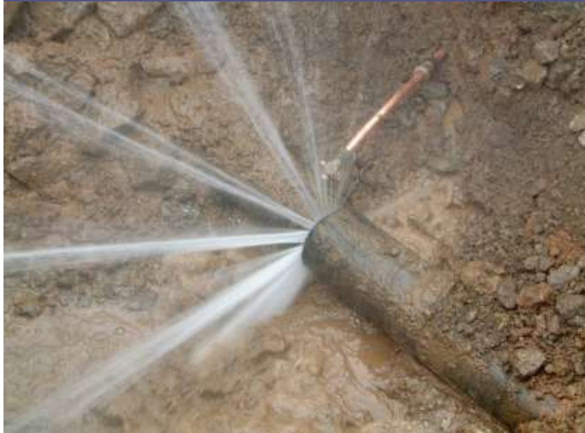
High-Pressure Leak
