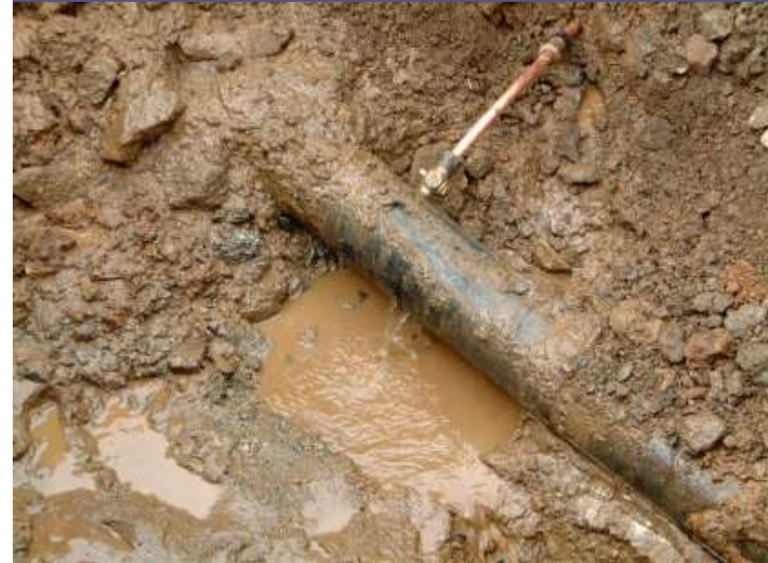
Low-Pressure Leak
