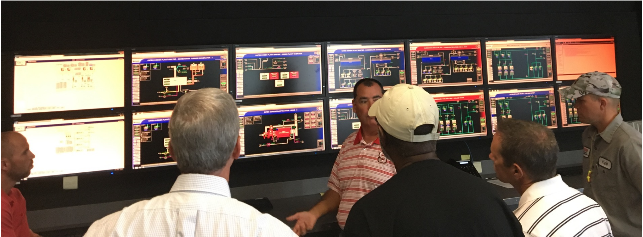
Two groups of Shaw operators visited NC State University's 11 MW CHP Plant to gain knowledge from the operations staff
