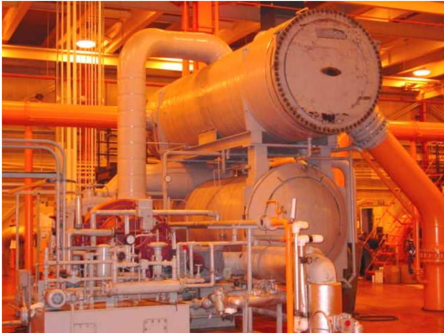
4,000 RT Steam Turbine Driven Chiller
