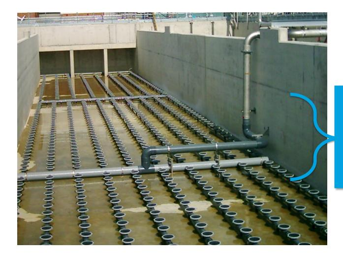
Distance from diffuser to water surface in feet divided by 2.31 = minimum header pressure in PSIG to form a bubble.
