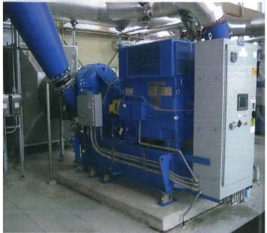
A dual-vane control blower can increase turndown capability. Tetra Tech
