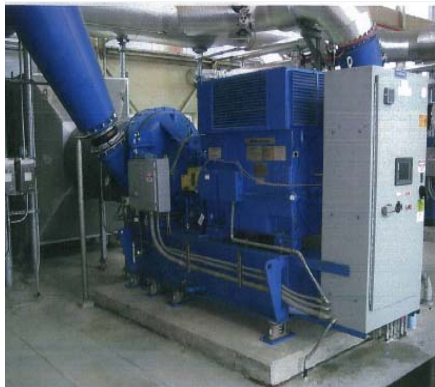
A dual-vane control blower can increase turndown capability. Tetra Tech
