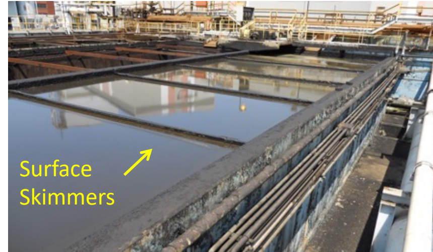
Settling/Separation tanks (chemical treatment)
