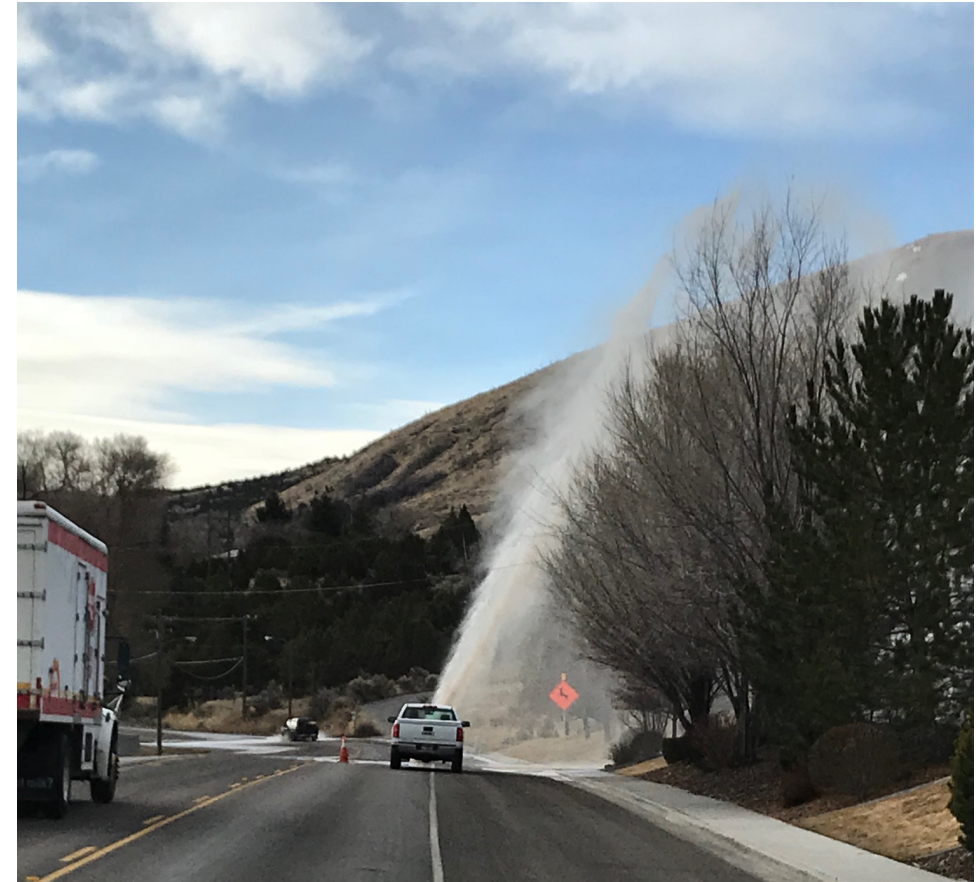
Leak on 12" main. Photo courtesy of Harold Hargaves, City of Pocatello, ID.
