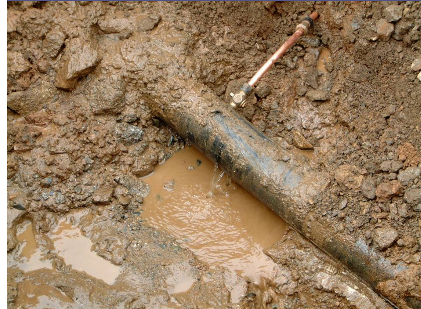
Low-Pressure Leak
