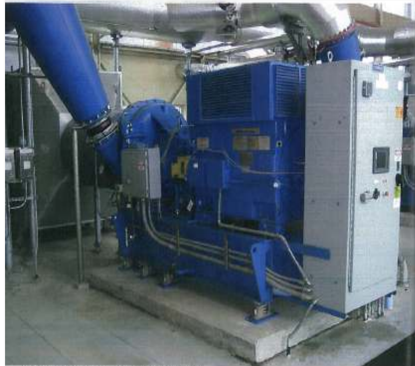
A dual-vane control blower can increase turndown capability. Ista Tech
