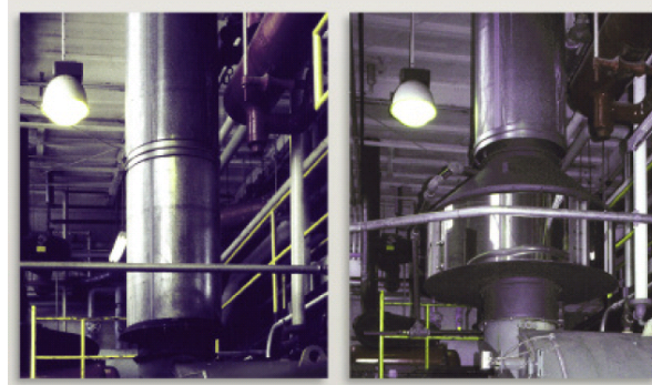
Example of use of economizer Before and after case (courtesy Cane Industries)
