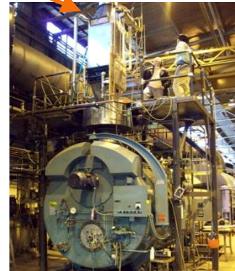
Super boiler that offers ~95% efficiency Before and after case (courtesy GTI)
